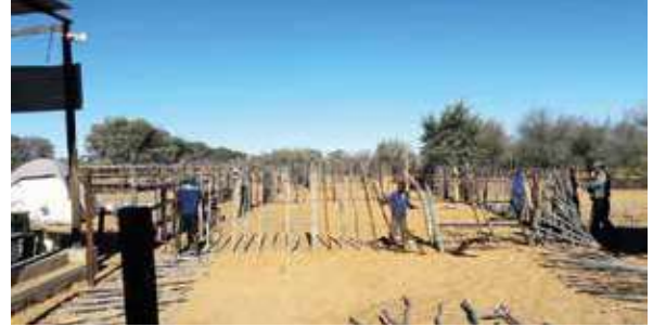
The old crush pen (left) before the construction of the new EU-compliant pen (right).
